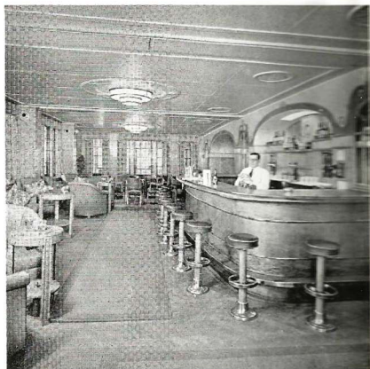
Strowgerphone installation aboard a luxury liner.
