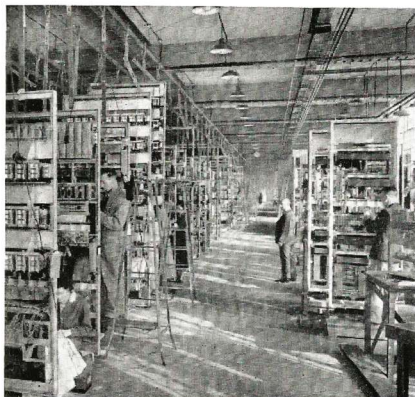
The rack wiring department.
